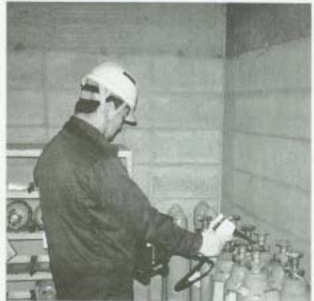
Leakage measurement from cylinder valve
