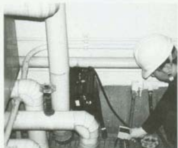
Solvent measurement of drainage pit.
